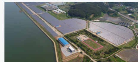
Seosan PV power plant
