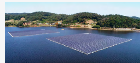
Owl Reservoir floating PV plant
