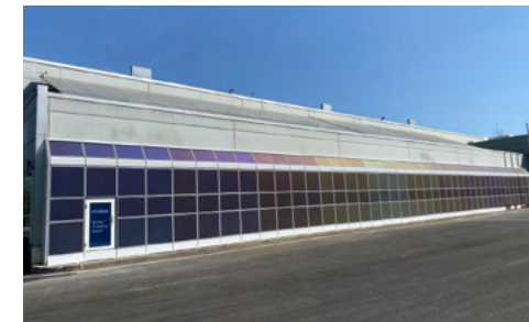
BIPV solution installed within the Eumseong Factory site
